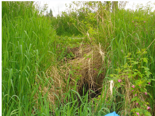
4 ↓ Existing Outlet Culvert to Nicomekl River
