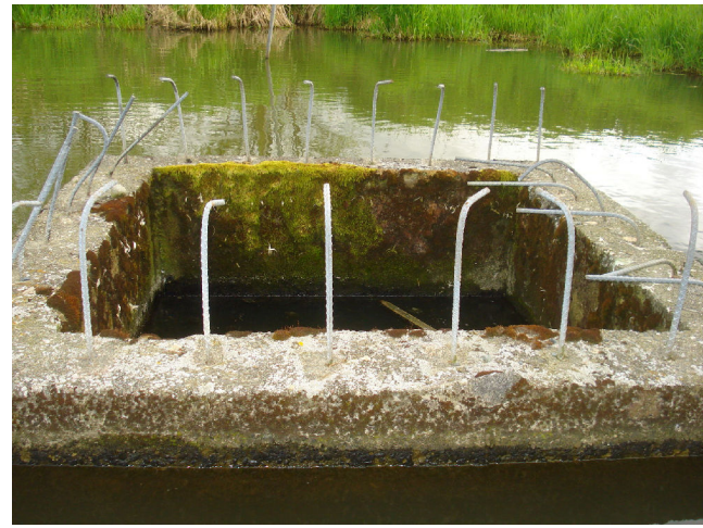
2 ↓ Abandoned Overflow Structure
