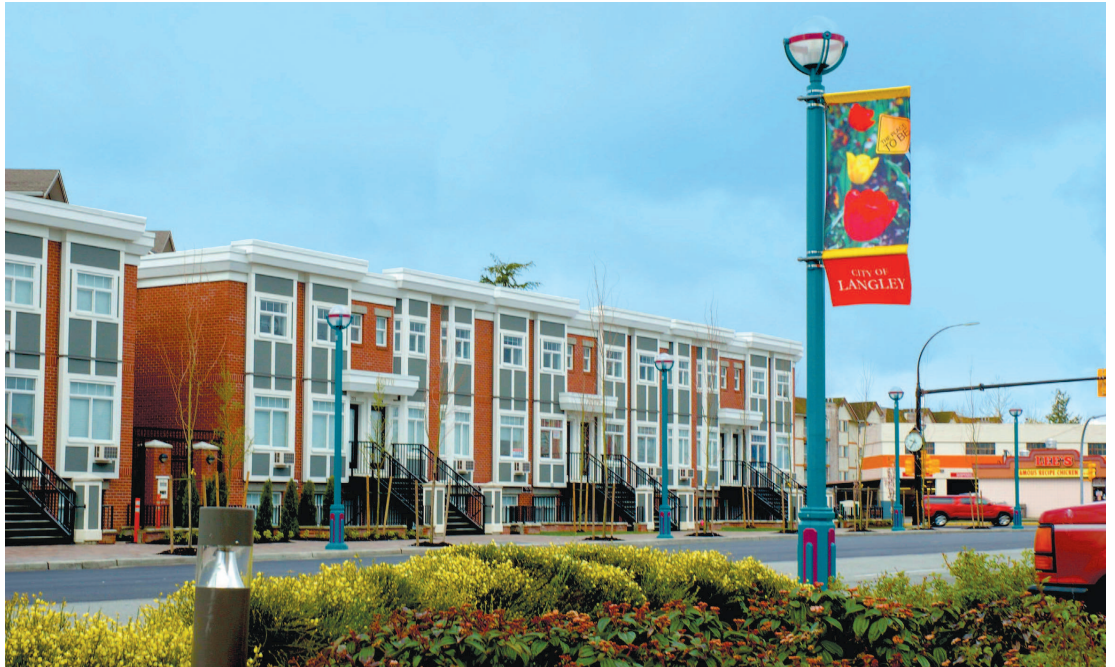
The multi-million Paddington Station Project transformed a previously contaminated old industrial site into an attractive multi-family residential project in the pedestrian-oriented downtown core.
